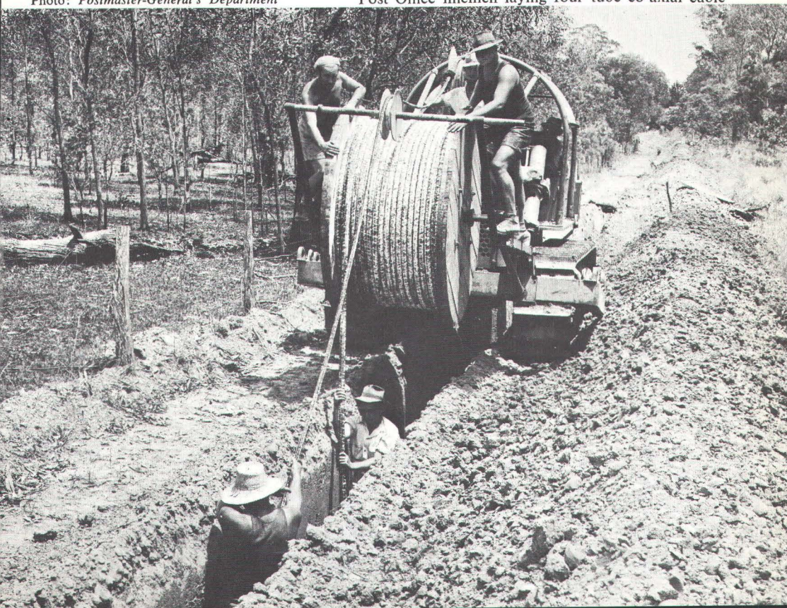
COMMUNICATION—Chapter 8 Post Office linemen laying four tube co-axial cable
